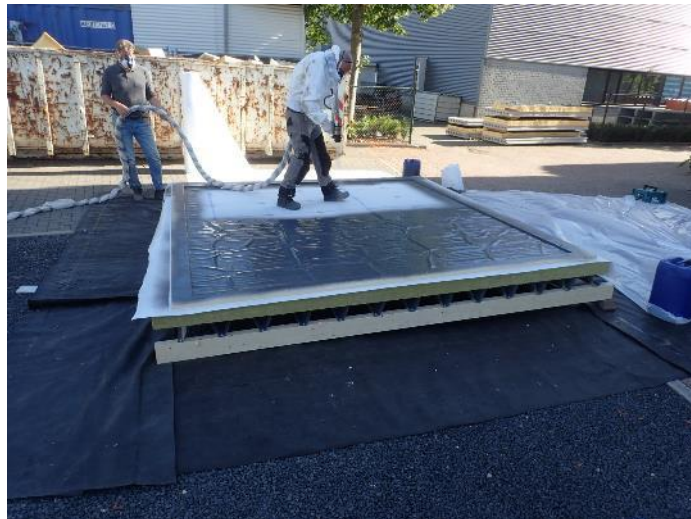
Photo 5 The coating is applied.
