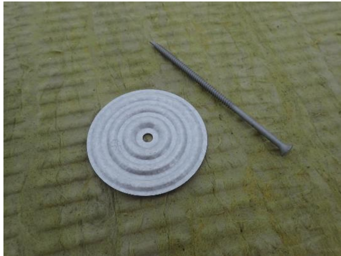
Photo 4 Detail of the fastening system.
