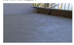
In order to level the surface after removing the tiles, **Rayston Level 503** was applied. The self-levelling support preparation mortar is a good choice if you need to turn a rough and uneven support into a levelled, well prepared surface, ready to support all following system layers.
