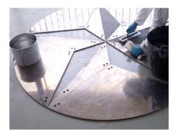
As a special decorative element, a metal mold was used on the terrace in Salou to form the design of a star, with a 2m diameter.
